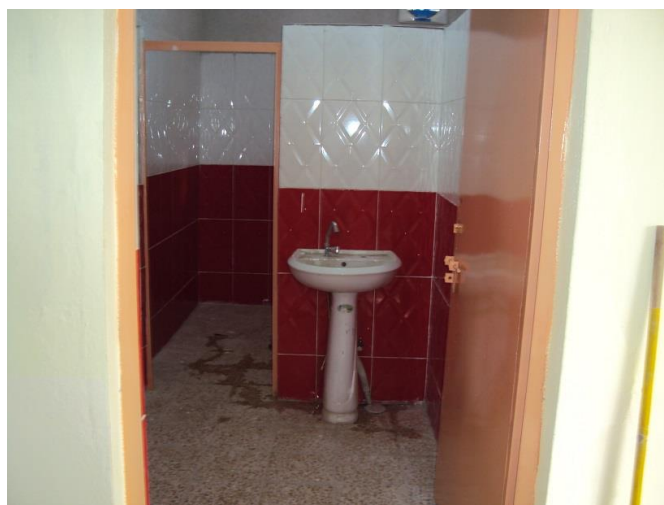
Above: A newly renovated bathroom facility in the Om Salama Intermediate School for Girls.
