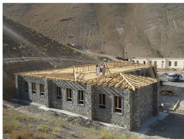
Above: Construction of the school
