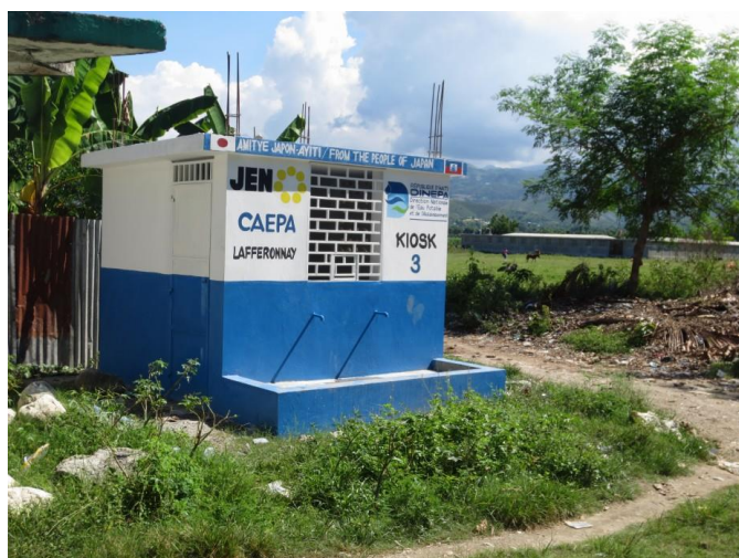
Above: One of many kiosk style water stations
