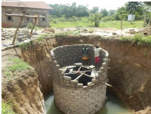
A new well is constructed by JEN
