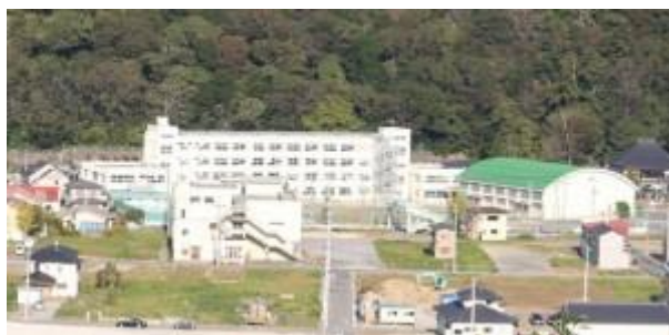
A school was finished restoration work
