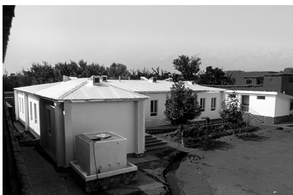
Above: The newly constructed Qalai Nasro Boys Middle School in Bagram.
